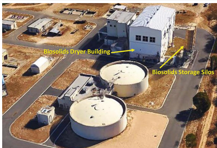
Figure 2. Class AA biosolids dryer and storage facilities, Tallahassee, FL. Credits: Map data ©2015: Google, DigitalGlobe
