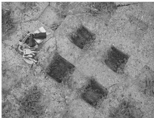
Fig. 3. Simulated maintenance on CGP surface
